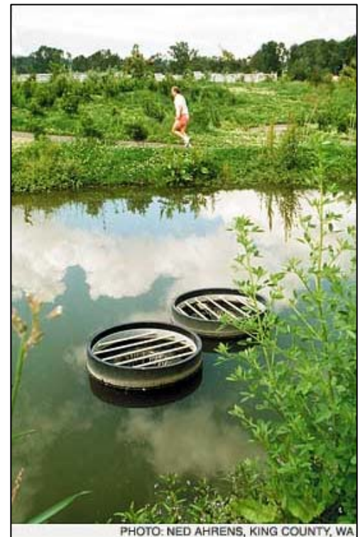
Stormwater management facility with recreational amenities.
